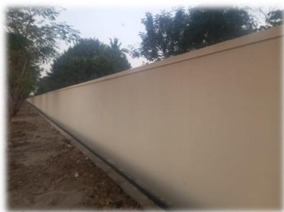
Compound Wall Works -Wipro
