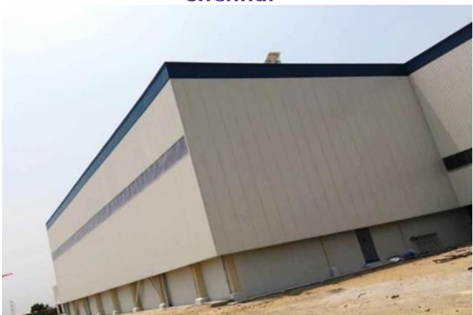
Ashok Leyland Technical Centre - Chennai
